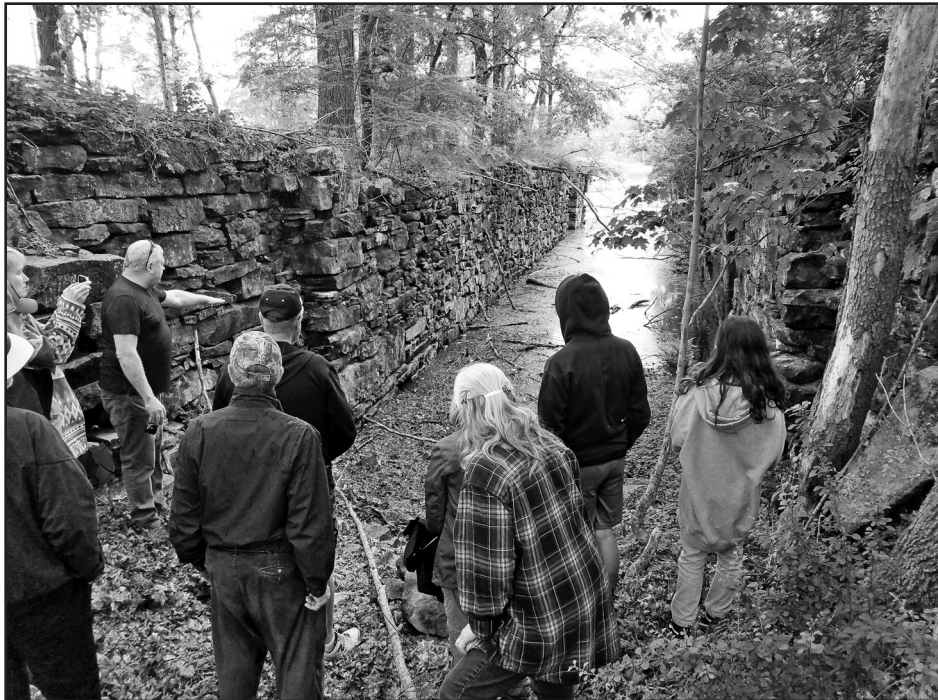
CANAL REMNANTS: D&H Transportation Heritage Council Vice-President Cliff Robinson, Jr. far left, points out extant features of the old Delaware & Hudson Canal Lock 41 near Phillipsport, NY during a May 20 bus tour that started in Port Jervis to trace a portion of the 108-mile boat transportation system that operated from 1828-1898 from Honesdale, PA to Eddyville, NY. Many of its hand-laid stone walls have stood the test of time. (Contributed Photo by Frank Coviello)
