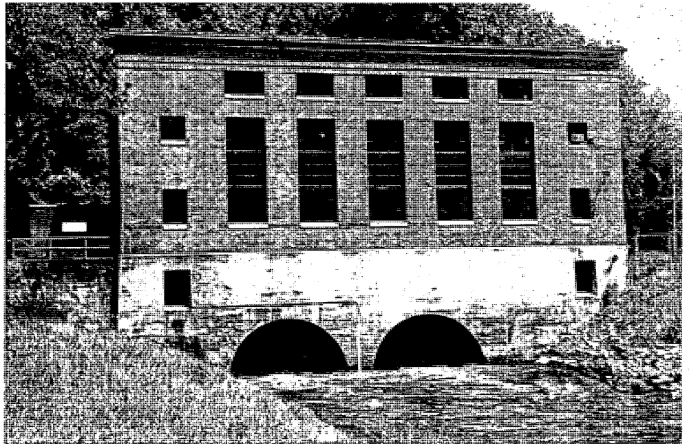
The Rio Hydroelectric Project. Orange and Rockland Utilities recently received a 30-year license to operate this and other hydropower facilities on the Mongaup River. Photo by Dave Soete.
