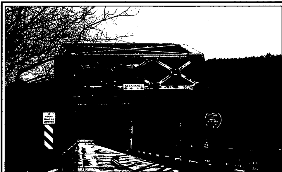
NEW BRIDGE COMING: The Pennsylvania Department of Transportation issued a Notice to Proceed with the design-build contract for a new Shohola-Barryville Bridge to the Fahs Rolston Paving Corp. of Binghamton on Feb. 12. A groundbreaking ceremony took place on March 25. The existing 1941 bridge which connects NY Route 55 with PA Route 434, pictured above, will be replaced with a 52-foot-wide, five-span bridge at a slightly northern location. The new $9.377 million bridge will have some unique design features based on public input, including a faux-bluestone concrete finish and a series of historical plaques in balconies along the pedestrian walkway. Traffic is expected to continue without interruption throughout the construction period, according to PENNDOT Project Manager Carla Medura. The targeted completion date is September 2006. Project updates may be requested from PENNDOT Community Relations Manager Dave Krisanda at (570) 963-4044 or dkrisanda@state.pa.us . (Photo by Laurie Ramie)
