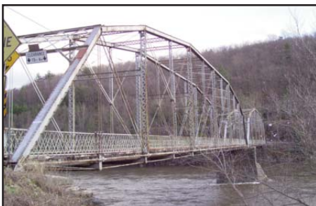
Pond Eddy, NY-Pond Eddy, PA Bridge
